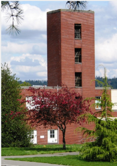
Building 18 & Hose Drying Tower
